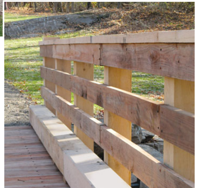
Figure 5. Native red oak 6x6 and 8x8 posts were attached to the predrilled brackets along the sides of the bridge, then the pressure-treated rail was attached. Wood planking and an oak curb completed the project.
