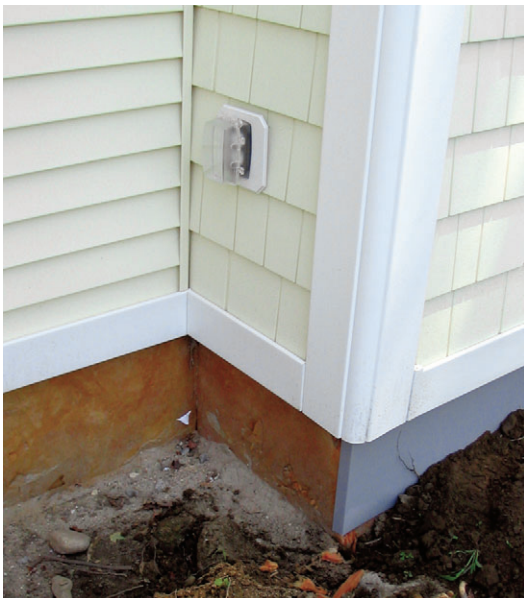
Figure 4. The siding contractor covered the exposed portion of the insulation board with vinyl coil stock. He waited until the job was nearly complete so that the vinyl wouldn’t get damaged by the work in progress.
