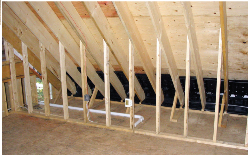
Figure 7. In an effort to prevent windwashing of attic insulation, the author first tried using cardboard baffles above the top plates, then stuffed the gaps between the baffles and the polystyrene ventilation chute with fiberglass batts (left). His discovery of a plastic baffle called AccuVent (below) made this process much easier.
