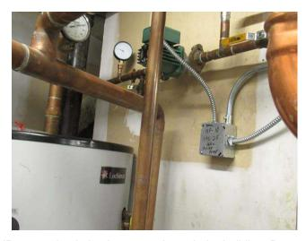
Component budget covers 1/2 HP pump circulating hot water through the building. Pump was replaced in 2018, per service contractor.
