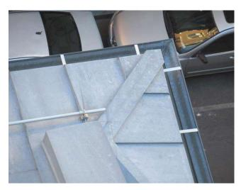
Component budget covers gutters and downspouts installed along front cornice and roof mechanical penthouses. Gutters and leaders are galvanized steel. Gutters and downspouts were in good condition during site visit.
