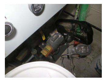
Component budget covers automatic fuel oil transfer pump and control panel. No reported operating issues. Area around pump and tank should be kept clear and not used for storage.
