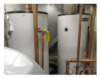
Component budget covers 119 gallon indirect domestic water heater tank installed in 2019. Useful life typically 10-15 years, depending on city water quality. Based on original tanks failing in 9 and 11 years, useful life set at 10 years.
