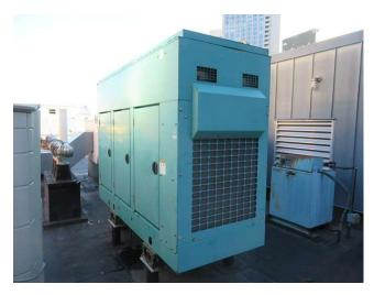
Component covers Cummins generator and peripheral equipment. Diesel-powered generator is rated at 200 kW. Generator was in good condition at site visit.
