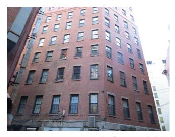
Component budget covers initial sealant and minor masonry repairs. Repairs typically include repointing damaged areas and sealing penetrations. Cleaning and sealing brick surface may also be required. Ongoing minor repairs are covered by separate component.
