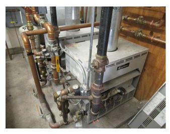
Component budget covers Lochinvar CWN270PM standard-efficiency boiler installed at initial construction providing domestic hot water for building through indirect water heater tanks listed separately.
