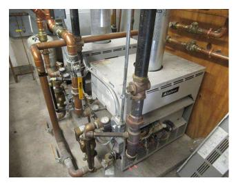
Component budget covers Lochinvar CWN270PM standard-efficiency boiler replaced in 2019. Boiler provides domestic hot water for building through indirect water heater tanks listed separately.
