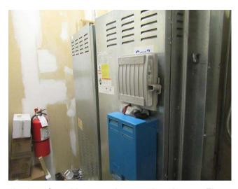
Component budget covers modernization of machine room-less traction elevator. Elevator was functioning normally at site visit. Since there is no machine room, elevator mechanical machine is located at top of hoistway and was not accessible during site visit.
