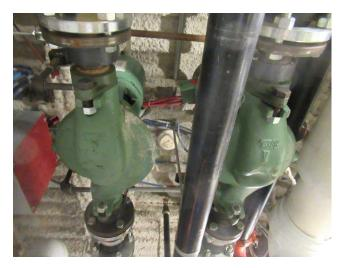
Component budget covers (2) circulation pumps for boiler water. In winter, boiler water is fed into condenser water loop with valves that control the temperature of the condenser water to 68F. Condenser water circulates to unit heat pumps.
