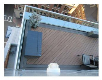
Component budget covers exterior terrace decks with composite or wood deck boards. Monolithic decks are non-structural and installed on sleepers over membrane roof. Terrace decks were not accessible during site visit. Decks have various types of decking installed.
