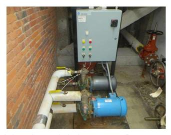
Component budget covers Thrush domestic water duplex booster pumps. Pumps are powered by 7.5 hp motors. Cost from similar association includes vertical removable-bladder hydropneumatic pressure tank.
