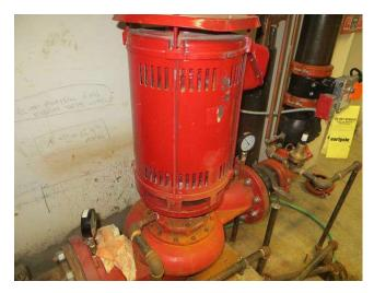
Component budget covers replacement of 50-HP fire pump & controller. No issues reported. Useful life extended to reflect pump rebuild component listed separately.
