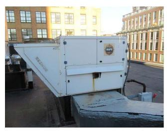
Component budget covers rooftop unit (RTU) providing heating and cooling for hallways. Unit also provides 100% ventilation/fresh air to building.
