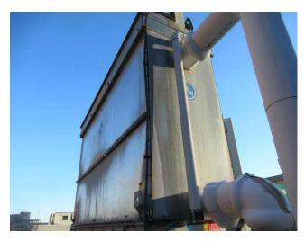
Component budget covers replacement of cooling tower which provides chilled water for building cooling. Condenser water circulation pumps are a separate component.
