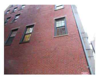
Component budget covers minor masonry repairs starting in 2024. Repairs typically include repointing damaged areas and replacing sealants to maintain water resistance. Cleaning and sealing brick surface in targeted areas may also be required. Major repairs are covered by separate component.
