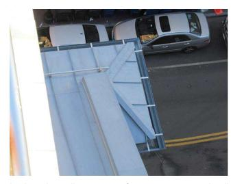
Component budget covers galvanized steel standing seam roofs, parapet caps, and wall panels. Unpainted galvanized steel appeared to be in good condition at site visit. No leaking issues reported.
