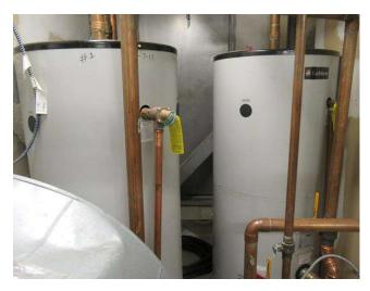
Component budget covers 119 gallon indirect domestic water heater tank installed in 2017. Useful life typically 10-15 years, depending on city water quality. Based on original tanks failing in 9 and 11 years, useful life set at 10 years.
