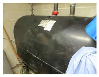
Component covers 275 gallon diesel fuel storage tanks located in basement storage room. Steel tank holds fuel for backup generator. No major issues reported. Tank may be without cathodic protection, but fuel usage is low so introduction of water in tank with fuel deliveries should be low also. Cathodic protection should be considered. Useful life increased from 30 to 35 years to reflect low refill frequency.
