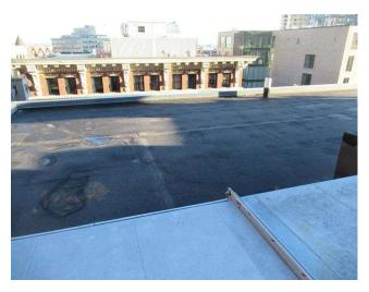
Component budget covers EPDM membrane roofs on building. EPDM is an extremely durable synthetic rubber roofing membrane (ethylene propylene diene terpolymer) widely used in low-slope ("flat" roof) buildings.
