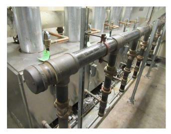
Component budget covers (5), HydroTherm MultiTemp, standard-efficiency (80%) boilers installed at original construction. Boilers provide hot water for building space heating.
