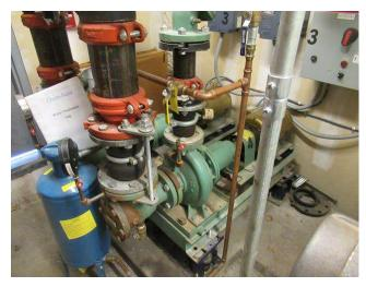
Component budget covers (2) circulation pumps for condensor water loop supplying hot and cold water to unit and common heat pumps. No issues reported by management. Pumps and motors appear original to construction. Variable frequency drives (VFDs) are used for soft start of motors to extend pump & motor life. There is no controller so pumps operate at a constant speed/flow. Useful life for pumps extended to to account for VFDs.
