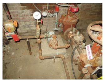
Component budget covers fire sprinkler jockey pump. Pump maintains wet sprinkler pipes at approximate target pressure to aid in sensing if a sprinkler head discharges. Jockey pump eliminates need for main fire pump to run to maintain system pressure. If sprinkler system has low leak/loss rate, pump may only run once a week.
