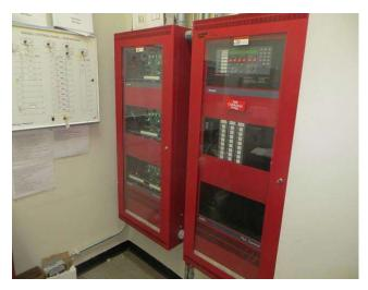
Component budget covers main parts of fire alarm system. The fire alarm system is composed of main fire alarm panel, smoke control panel and fire annunciator. Component does not include re-wiring, pull stations, fire emergency lights, heat detectors, or horns. Replacement of peripheral devices is currently done on an as-needed basis. Funding for these devices can be added if desired.
