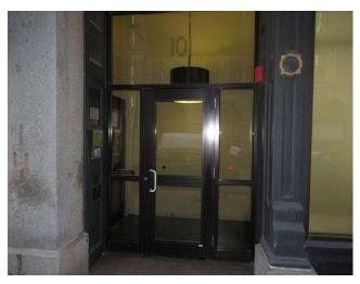
Component budget covers exterior aluminum frame full view commercial main entry door. Door was in good condition during site visit with no issues reported by client. Door is protected by awning and recessed into building. The remaining life of this component has been extended due to its condition at our most recent site visit.
