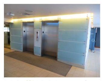
Component covers combined modernization of Otis hydraulic elevator systems for two elevators.
