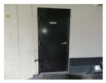
Component covers five exterior fire doors to parking garage. Two doors were replaced in 2016 per client for \$1900 per door. 2010 used as average placed-in service date for budgeting purposes.
