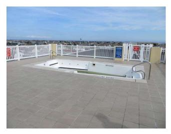
Pool access from north stair is protected by aluminum fence. Fence was in good condition during site visit. Component covers complete replacement of fencing. No quantity is listed in prior reserve study.
