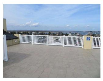
Pool access from south stair and pool area are protected by vinyl fence. Fence was in good condition during site visit. Component covers complete replacement of fencing. No quantity is listed in prior reserve study.
