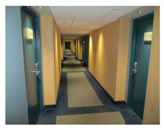
Component cover replacement of corridor light fixtures only. Replacement with LED fixtures being considered by client. Current fixtures have non-standard lamp base.
