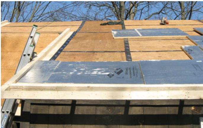
Figure 1. To accommodate the extra thickness of the exterior wall insulation, the author extended the roof overhangs with dimension lumber (above left and above). Doubled 2x4s along the edge of the rake (left) will capture the double layer of 1½-inch foam board to be installed on the roof. Note the spray foam used to seal gaps in the roof sheathing.
