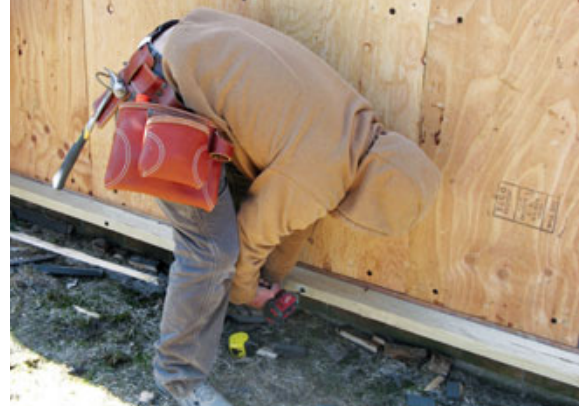
Figure 3. After installing a layer of \frac{3}{4} -inch plywood over the existing barnboard, the author sealed the critical wall-to-roof juncture with flashing tape, spray foam, and a rubber gasket (above left). A 2x4 ledger at the base of the wall (above) temporarily supported the double layer of 1-inch rigid foam, which was lapped at the corners (left), carefully cut in at the soffit, and sealed to framing members with spray foam (below).
