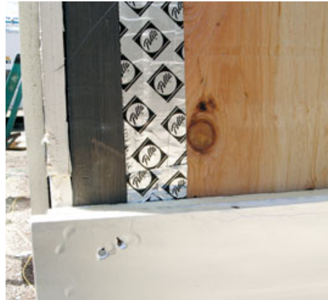
Figure 3. After installing a layer of \frac{3}{4} -inch plywood over the existing barnboard, the author sealed the critical wall-to-roof juncture with flashing tape, spray foam, and a rubber gasket (above left). A 2x4 ledger at the base of the wall (above) temporarily supported the double layer of 1-inch rigid foam, which was lapped at the corners (left), carefully cut in at the soffit, and sealed to framing members with spray foam (below).
