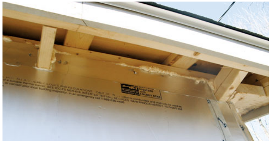
Figure 3. After installing a layer of \frac{3}{4} -inch plywood over the existing barnboard, the author sealed the critical wall-to-roof juncture with flashing tape, spray foam, and a rubber gasket (above left). A 2x4 ledger at the base of the wall (above) temporarily supported the double layer of 1-inch rigid foam, which was lapped at the corners (left), carefully cut in at the soffit, and sealed to framing members with spray foam (below).
