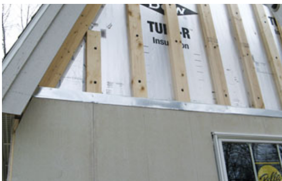
Figure 4. Once the joints in the outer layer of rigid foam had been taped, the crew installed vertical 2x4s on 16-inch centers (top left), then set the windows, flashing them to the plane of the furring members. Site-bent flashing taped to the foil-faced foam protects the window heads (top right). HardiePanels were nailed to the furring and Z-flashed at horizontal joints (above left). Rough-textured Miratec was used for trim (above right).
