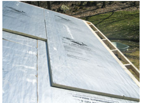
Figure 2. The crew sealed the original roof sheathing with flashing tape (above left), then installed two layers of rigid foam, staggering the seams (above) and taping the joints in the top layer (far left). A new layer of roof sheathing was installed over 2x4 battens, with gaps at the top for ridge venting (left).
