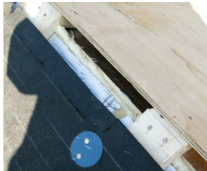
Figure 2. The crew sealed the original roof sheathing with flashing tape (above left), then installed two layers of rigid foam, staggering the seams (above) and taping the joints in the top layer (far left). A new layer of roof sheathing was installed over 2x4 battens, with gaps at the top for ridge venting (left).
