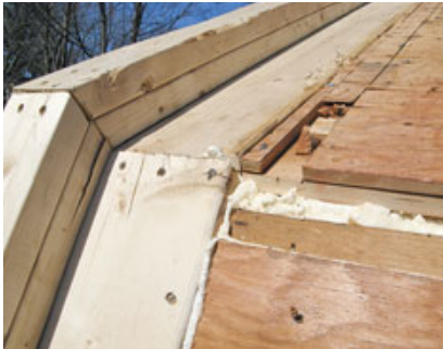
Figure 1. To accommodate the extra thickness of the exterior wall insulation, the author extended the roof overhangs with dimension lumber (above left and above). Doubled 2x4s along the edge of the rake (left) will capture the double layer of 1½-inch foam board to be installed on the roof. Note the spray foam used to seal gaps in the roof sheathing.
