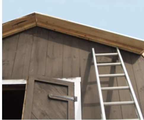
Figure 1. To accommodate the extra thickness of the exterior wall insulation, the author extended the roof overhangs with dimension lumber (above left and above). Doubled 2x4s along the edge of the rake (left) will capture the double layer of 1½-inch foam board to be installed on the roof. Note the spray foam used to seal gaps in the roof sheathing.
