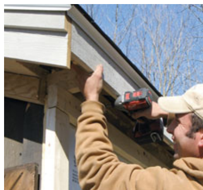
Figure 4. Once the joints in the outer layer of rigid foam had been taped, the crew installed vertical 2x4s on 16-inch centers (top left), then set the windows, flashing them to the plane of the furring members. Site-bent flashing taped to the foil-faced foam protects the window heads (top right). HardiePanels were nailed to the furring and Z-flashed at horizontal joints (above left). Rough-textured Miratec was used for trim (above right).
