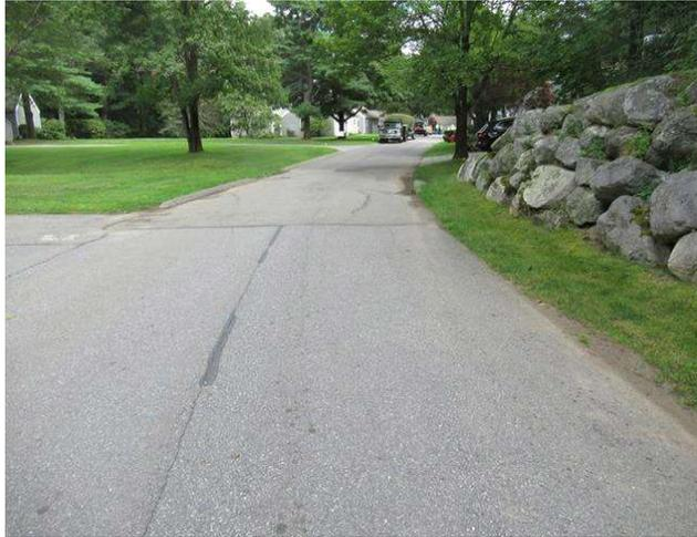
Component budget covers overlay of roadway asphalt road areas. Asphalt was replaced in 2009, per client. Asphalt is in generally good condition. Cracks and prior patch repairs evident during site inspection. Some cracks have been sealed. Driveways are listed separately. Differentiation between road and driveways not clear in some areas.
