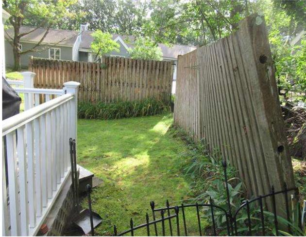
Component budget covers replacement of wood privacy barriers installed in side and rear yards of units. Each 6' tall fence is comprised of 1, 2, or 3 8' long sections. Total number of sections is 23 for a total length of 184'. Barriers were generally in poor condition. Some were leaning and should be repaired. Resetting, cleaning, and sealing wood fences could extend service life. Placed-in-service date per client.
