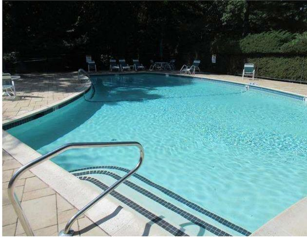
Component budget covers resurfacing pool plaster. Plaster surface, coping, water line tile, and skimmers were replaced in 2010, per client. Plaster surface was in good to fair condition at site visit. Remaining life extended to reflect condition.
