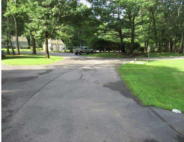
Component budget covers overlay of roadway asphalt road areas. Asphalt was replaced in 2013, per client. Asphalt is in generally good condition. Numerous cracks evident during site inspection. Most cracks have been sealed. Driveways are listed separately. Differentiation between road and driveways not clear in some areas.
