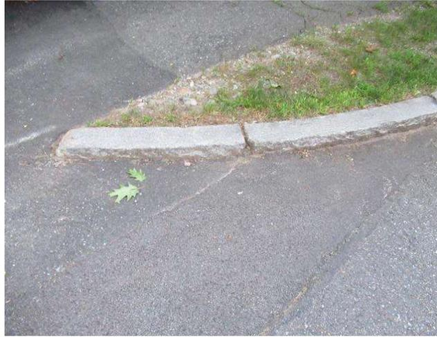
Component covers granite curbing on roadway areas. Curbs were in good condition during site inspection. No damage or displaced sections were observed. Component listed for inventory purposes.
