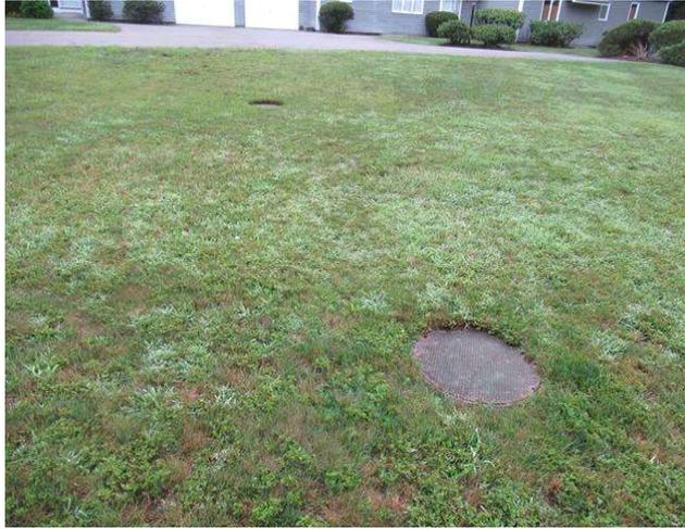
Component budget covers periodic replacement of concrete septic tanks and pump chamber tanks. Tank useful life is typically between 40 years and indefinite. No tank issues reported in Title V reports. A number of concrete distribution boxes have recently been replaced.
