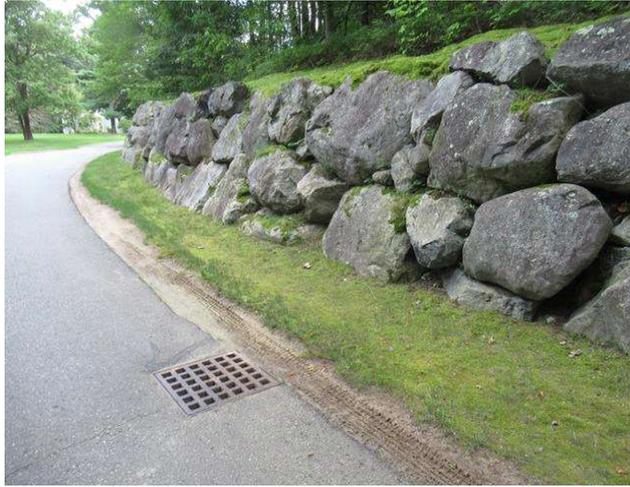
Component budget covers periodic repair and replacement of retaining walls around association. Walls were in generally good condition at site visit. Most walls were stone. A few walls were constructed from pressure-treated wood. Some wood retaining walls were leaning and decaying. Replacement of wood retaining walls will be required in near future. Walls should be evaluated annually and minor repairs funded by operating budget.
