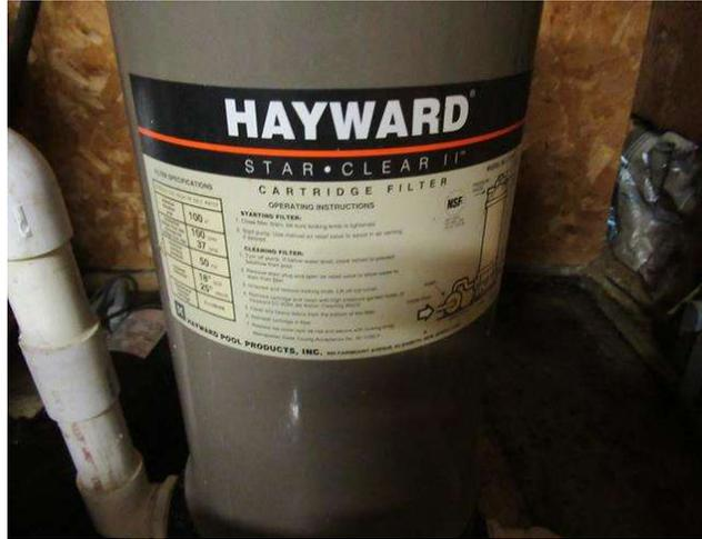
Component budget covers two cartridge pool filters. Filters appeared in good condition. No issues reported. Filters were installed in 1996, per client. The remaining life of this component has been extended due to its condition at our most recent site visit.
