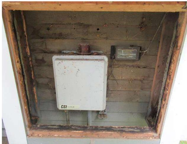
Component budget covers septic lift duplex pumps and controls. No information on pumps available. No issues reported. Pump useful life is typically between 10 and 15 years. Component assumes that one pump system is replaced every 4 years. Allowance should be revised, based on association experience, in future reserve study updates.
