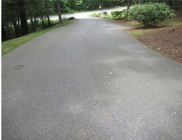
Component budget covers overlay of roadway asphalt road areas. Asphalt was replaced in 2011, per client. Asphalt is in very good condition. Numerous cracks and repairs evident during site inspection. Some cracks have been sealed. Driveways are listed separately. Differentiation between road and driveways not clear in some areas.
