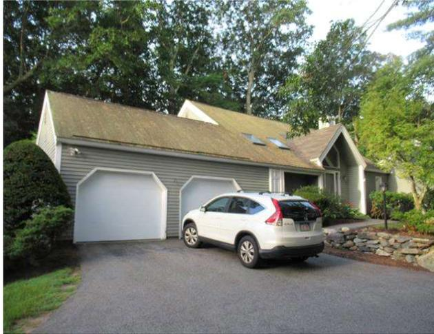
Component budget covers rebuild of asphalt driveways and parking areas. Asphalt is in generally good condition with some cracks observed. Roads are listed separately. Differentiation between roads and driveways not clear in some areas. See additional general comments listed under "Asphalt - Overlay, C".
