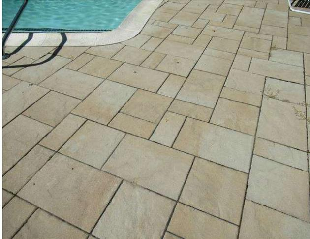
Component budget covers periodic partial re-setting of pool deck concrete pavers. Pool deck was in good condition. Some moss is growing in joints between pavers in shady areas. Paver deck was installed some time after 2015 prior reserve study that indicates poor concrete original pool deck. Irregular pool deck area measurement is approximate. Allowance should be revised, based on association experience, in future reserve study updates.
