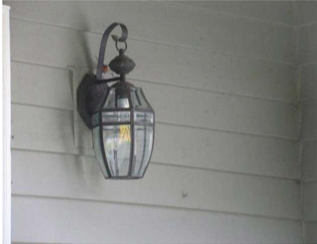
Component budget covers replacement of light fixtures on exterior of units. Fixtures are in generally good to fair condition. Lights are generally installed at exterior doors for each unit. Fixture type and location is inconsistent on some units. Approximate total used.
