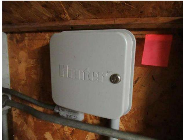
Component budget covers periodic allowance for partial replacement of irrigation system major components: controllers, backflow preventers & zone valves. An irrigation system is installed on each street. Systems on C and L use municipal water supply. Wells supply water for S and I. Allowance should be adjusted based on association experience.
