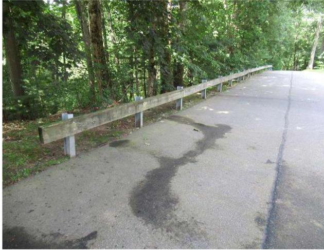
Component budget covers replacement of wood guardrail along roadway opposite S units 16, 17, & 18. Guardrail was in fair condition with one broken section in need of replacement. Several steel posts were leaning, but still generally functional. Wood rails will need replacement more frequently than galvanized steel posts. Useful life based on steel posts. Replace wood rails as needed from operating budget.
