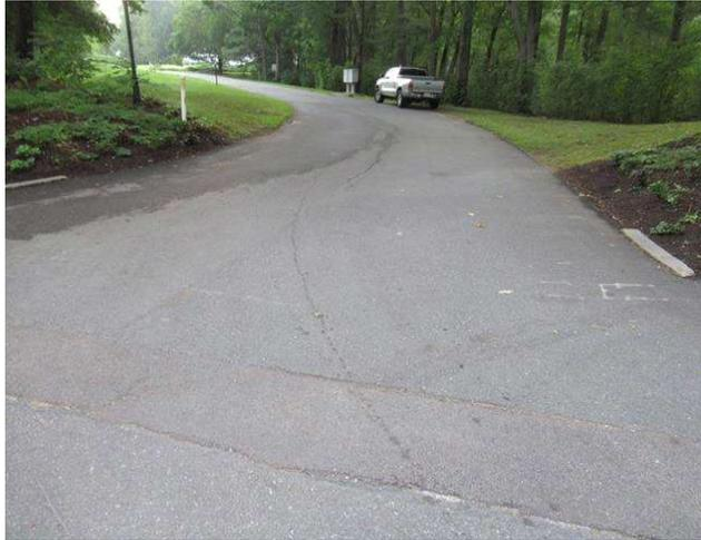
Component budget covers overlay of roadway asphalt areas. Asphalt was installed in 2016, per client, and is in good condition. Some cracks visible at site inspection. Cracks have not been sealed. Driveways are listed separately.
