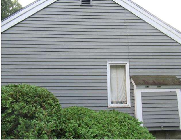
Component budget covers annual repairs of wood clapboard siding and trim on all buildings in association. Overall, siding was in good to fair condition at site visit. Buildings on I were in good condition after repairs and painting. Siding has basic trim details and is uniform throughout the association. Expected annual budget range of \$30,000 - \$40,000 provided by client.
