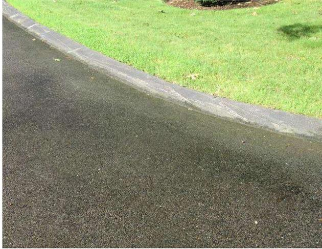
Component budget covers roadway asphalt berm/curbing. Asphalt berms were in generally good condition at site inspection. Some minor damage from plowing and other impacts were noted. Placed-in-service date for Steepletree asphalt project used.
