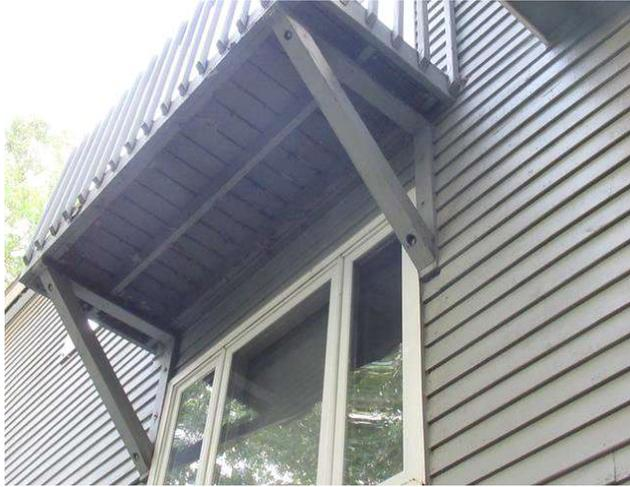
Component budget covers replacement of unit balcony structure only. Unit owners are responsible for railings and deck boards. There were originally 17 balconies, but 3 were replaced with sliding doors and railings by owners. Balcony structures appeared to be in good condition at site visit, but are nearing end of service life for framing. Balconies should be inspected in detail this year to ensure safety and confirm when replacements may be required.
