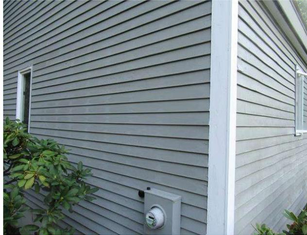
Component budget covers periodic major repairs of wood clapboard siding and trim on all buildings in association. Overall, siding was in good to fair condition at site visit. Siding has basic trim details and is uniform throughout the association. Pool house is included in I total.
