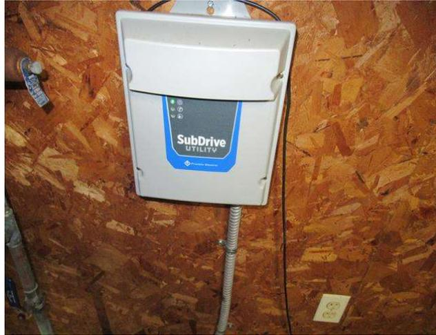
Component budget covers submersible well pumps and controls. Wells supply water for S and I. I well is powered by variable speed pump. The actual date this component was placed into service is not available. For budgeting purposes, this date is assumed to be 15 years after original well was drilled. Useful life increased to 20 years for variable speed pump. Allowance should be adjusted based on association experience.
