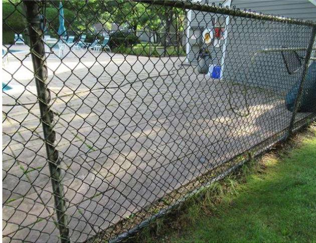
Component budget covers pool chain link fencing. Fencing was fair condition. Fence is functional, but paint is peeling/missing. Fence is original, per client. The remaining life of this component has been extended due to its condition at our most recent site visit.
