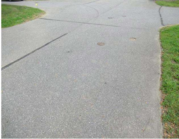
Component budget is for regular maintenance of asphalt areas before asphalt overlay. Three year cycle is recommended due to current pavement condition. Asphalt is in generally good condition. Some cracks and patches in asphalt were evident during site inspection. Most cracks have not been sealed. Component budget should be revised based on association experience as pavement ages.
